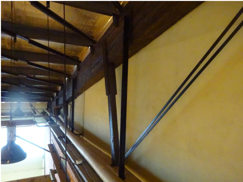
Klebebinder Achse 10/F-I
