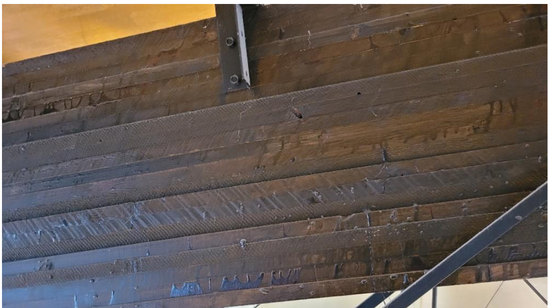
Klebebinder, b/h = \text{ca. } 100/640\text{ mm}
