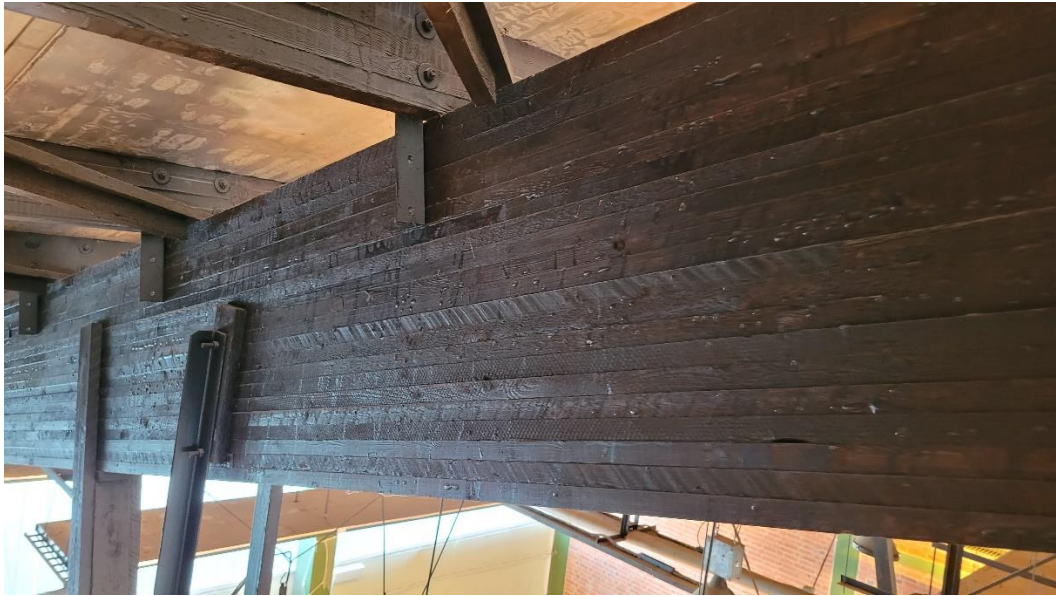
Klebebinder Achse 8/F-I
