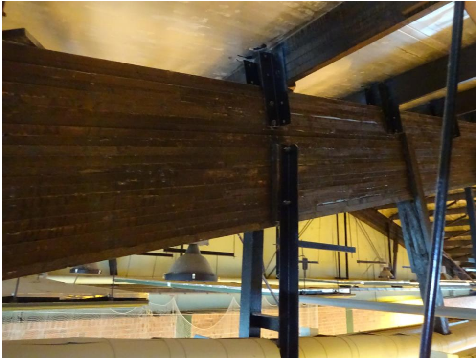
Klebebinder Achse 18/N-I
